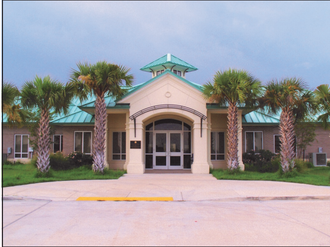
The Student & Faculty Housing Complex, which includes the Student Activities Center (pictured left), was opened in Spring 2010 on the Lake Campus (photo by Eddie Francis)
