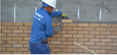
A worker lays bricks at Bashful Building
