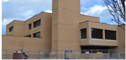
Flood gates to be installed at the University Center
