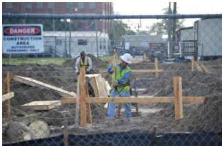
Workers lay the foundation of the Small Business Incubator
