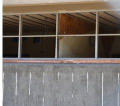
Window frames installed at Bashful Building
