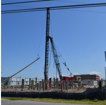
Signs — and sounds — of progress at Small Business Incubator site
