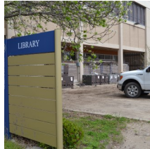
Brickwork outside of the Library is 99 percent complete
