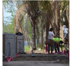
Workers lay sidewalk frames around the University Center
