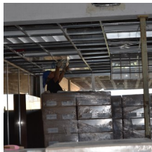
Workers install light fixtures in Library
