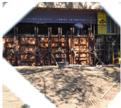
Floodwall around Bashful Building about 95% complete
