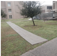
Temporary sidewalk installed
