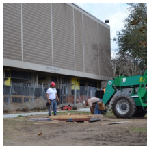
Workers build flood wall frame in front of Bashful Building
