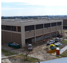
Bricklaying to start next week at Library
