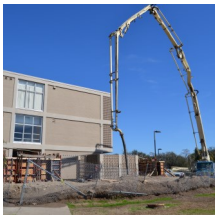
Cement poured for floodwall at Bashful Building
