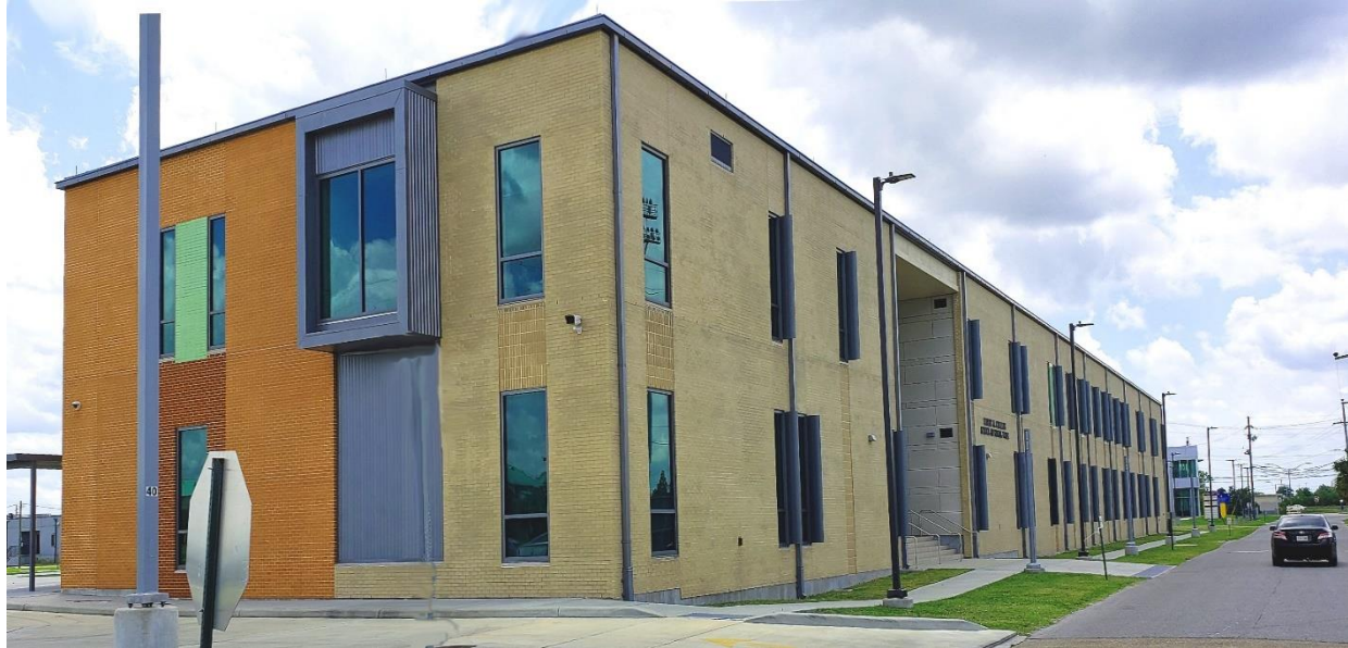
Millie M. Charles Social Work Building
